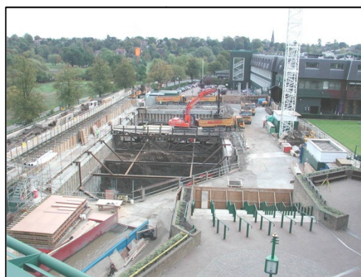
Basement Excavation – AELTCC Lawn Tennis Museum, Wimbledon
